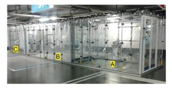
The unit contains three separate chambers with increasing negative pressure and unidirectional airflow.
